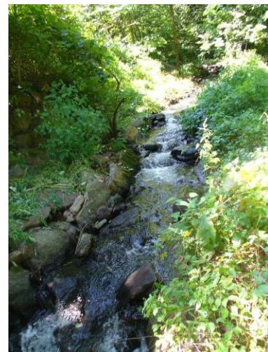
The lower portion of the Davis Pond Fishway, showing the nature-like channel that brings fish up from the base of the spillway to the exit, shown to the left.
