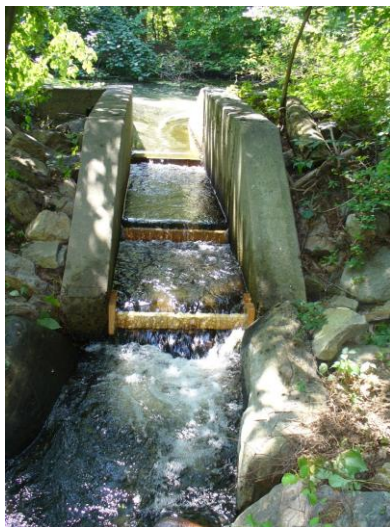
The exit of the Davis Pond Fishway, showing new wooden weirs. This section passes through the earthen dam.
